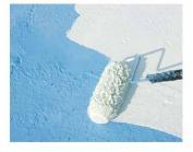
**OLYMPIC FUSION PLUS** — Converts your worn rubber-base coated pool to an epoxy finish. Clean your pool according the surface preparation instructions on the label, and roll on FUSION PLUS. Then follow with one coat of ZERON or two coats of POXOLON 2. Your rubber-to-epoxy finish will be beautiful and will last for many years.
