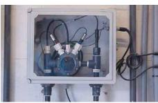
05-123 SENSOR CELL CABINET - Lockable fiberglass cabinet to protect probes. Includes: acrylic see-thru sensor cell. Houses Chemtrol ORP and pH probes and plumbing fittings. By-pass line assembly ordered separately.
