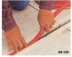
FOAM SEALANT BACKER - Polyurethane backer rod for expansion joints and between coping and cement deck.
